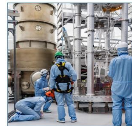
Figure 4: Installation works at ETpathfinder
